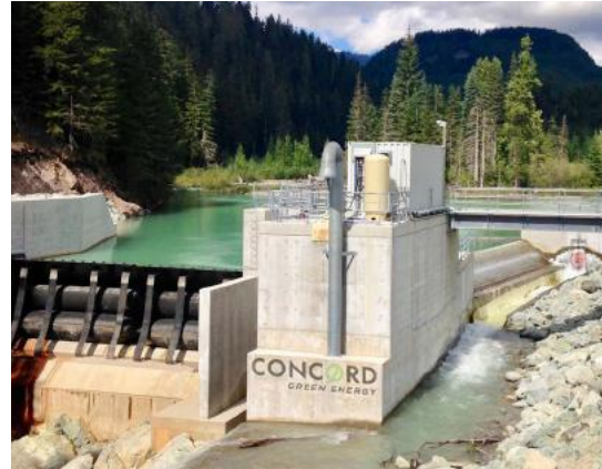
Skookum Power is a 25 MW run-of-river hydro-electricity project that will deliver clean renewable electricity to BC residents.
